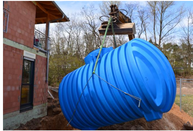
Regenwasserzisterne © Adobe Stock, Ilhan Balta
